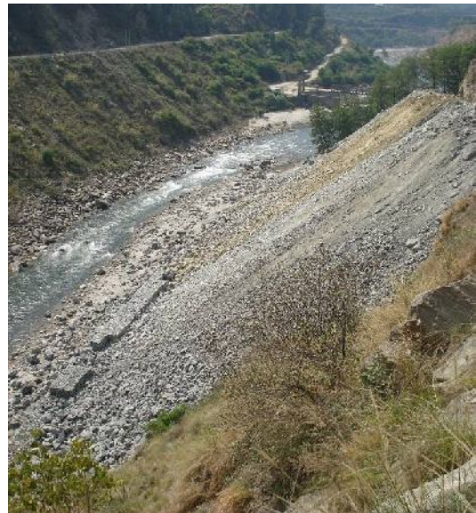
Photo-21& 22: Muck Dumping at Sawra Kuddu project site- violation of clearance conditions
