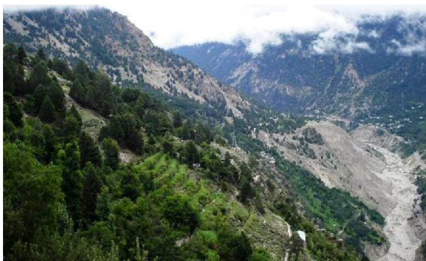
Photo-15: Khadra landslide – 3 separate tunnels are proposed on this already fragile mountain
