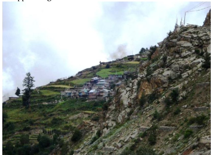
Photo-16: Loose rock outcrops below which Tokhtu village is located and tunnel of Kashang Stage-IV is going to pass
