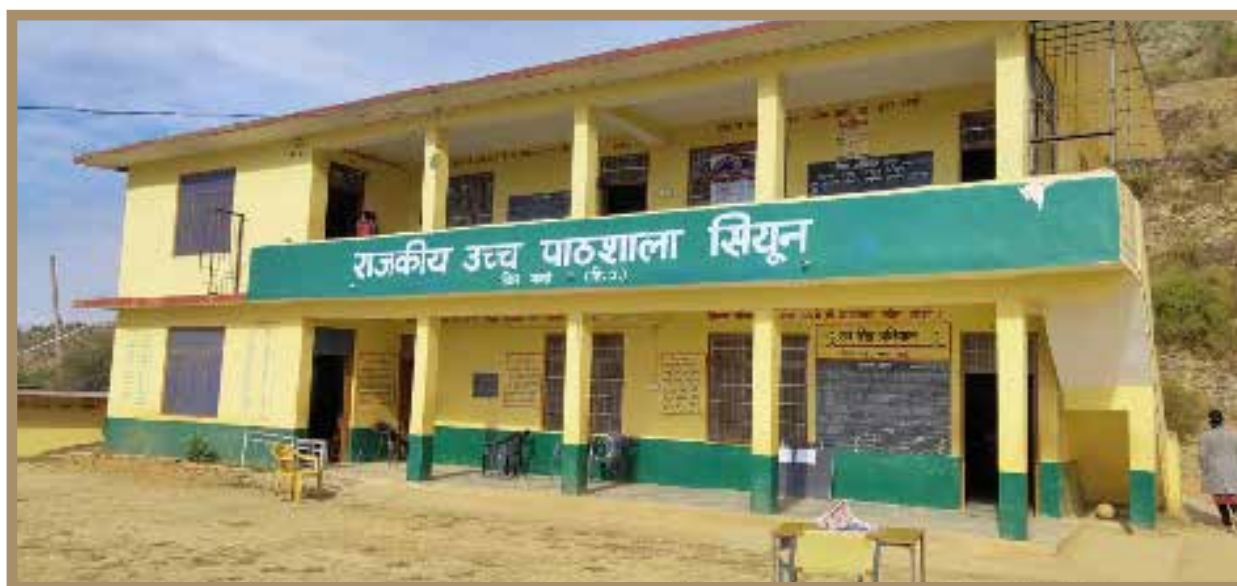
A school built in Siyun Panchayat back in 2008. The land was under the category of forest and involved no trees at the time as reported by the FRC. The FRC is now hoping the land will be diverted to the education department but the file is pending
